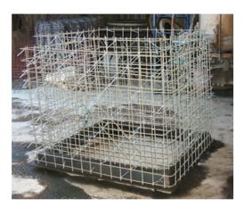
Fig. 2—A complete GFRP cage before concrete casting
